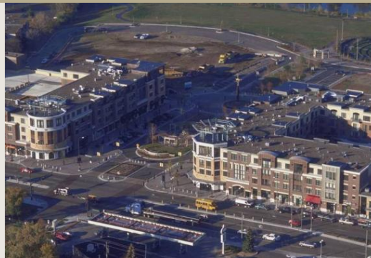
Corridor retrofit after
