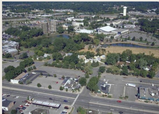
Corridor retrofit before
